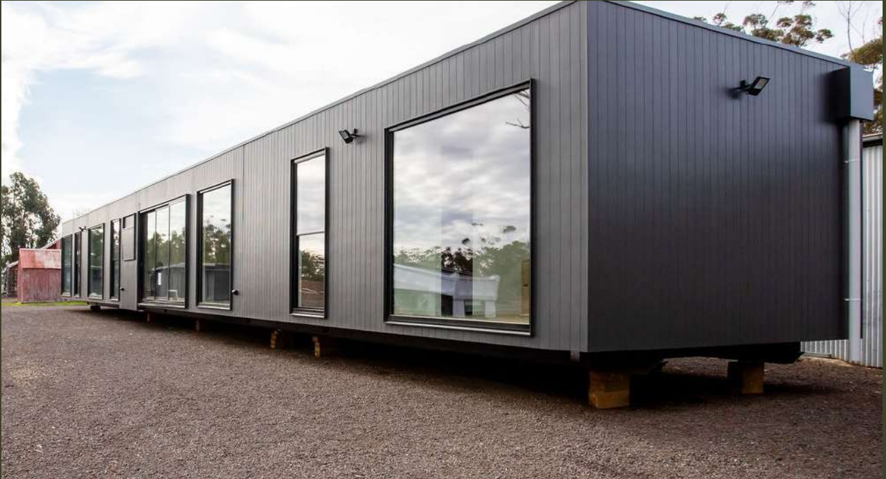
THE THREE MODULES AT HESSE
