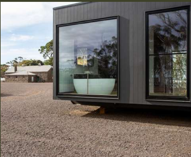
CLADDING AND GLAZING COMPLETE
